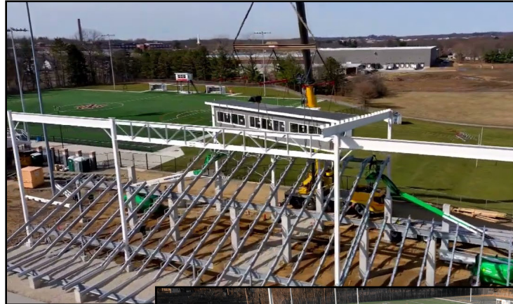
Top: The new pressbox being lifted into place on the new Grandstands.
